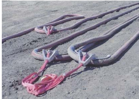
Multiple cables pulled with multiple grabs
