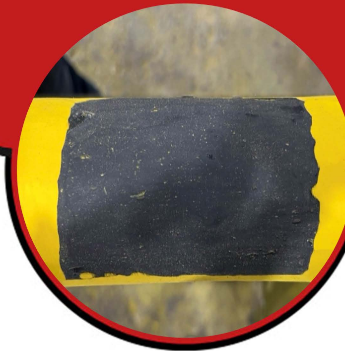
Completed Jacket Repair Patch
