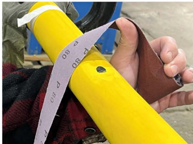
Prepare damaged jacket area
